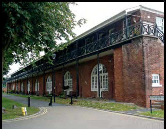
■ Higher Barracks, (CMRO) Exeter - now a housing estate Picture: Mr N Brown
