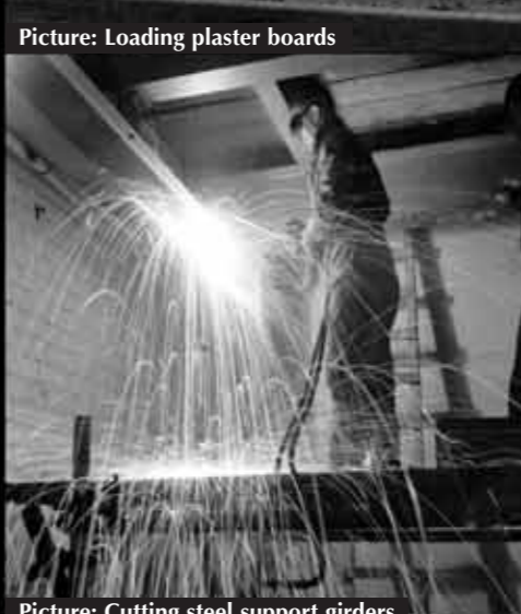
Picture: Cutting steel support girders
