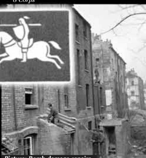
Picture: Bomb damage repairs
