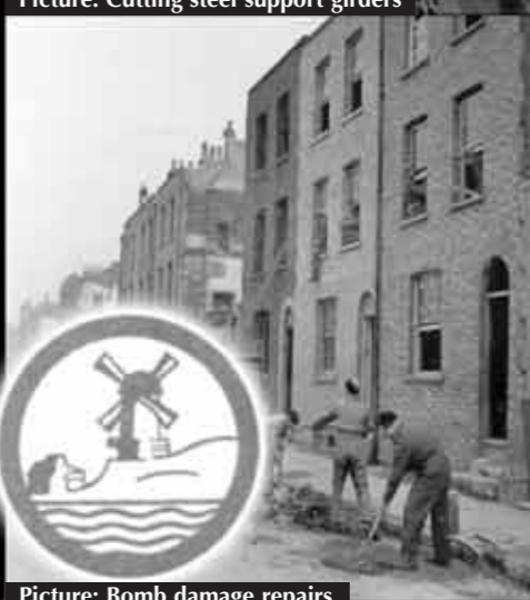
Picture: Bomb damage repairs
