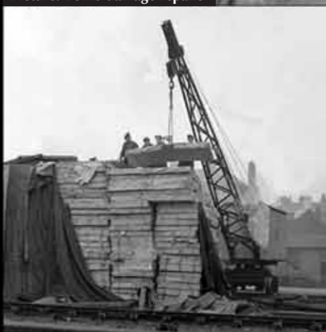
Picture: Loading plaster boards
